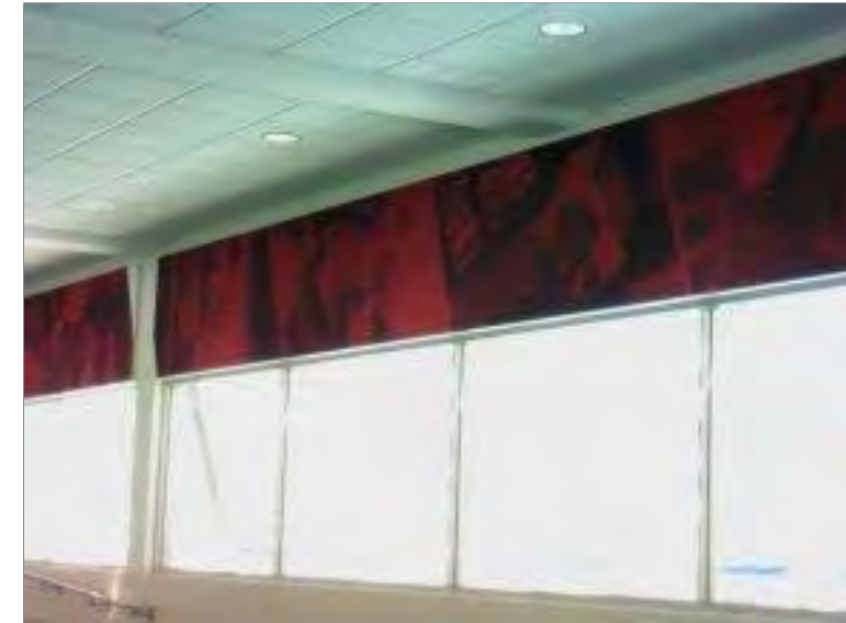
Photo 75: Digital image of the curtainwall systems throughout the Concourse area.
