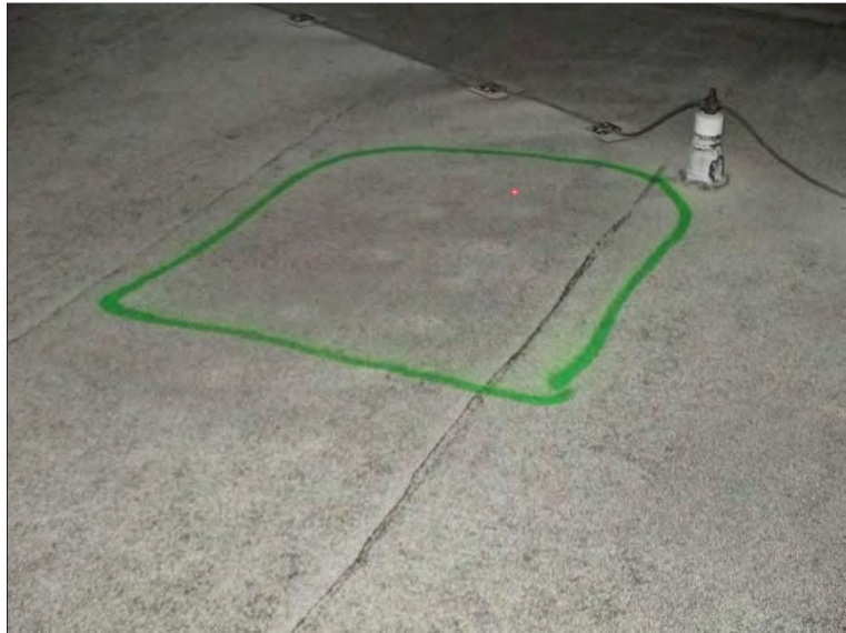
Photo 11: Overview of Thermogram #11 location at Roof #16.
