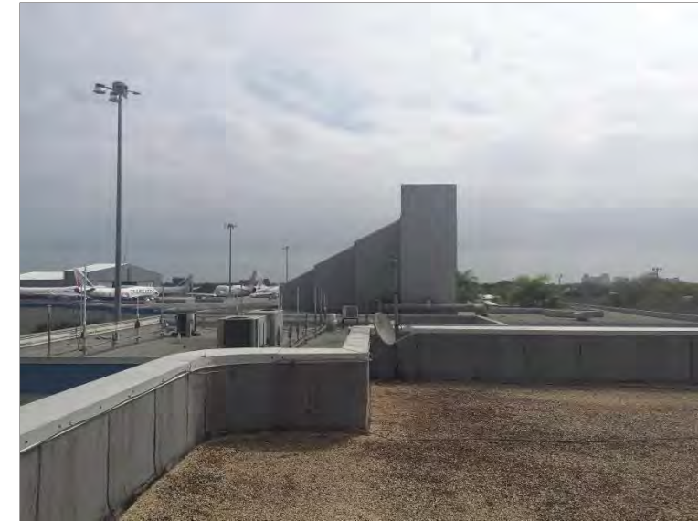
Photo 19: Overview of roof areas 12, 13 and 14.
