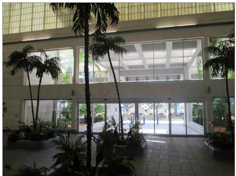
Photo 26: Interior view of window assemblies in the Atrium area throughout the south elevation.
