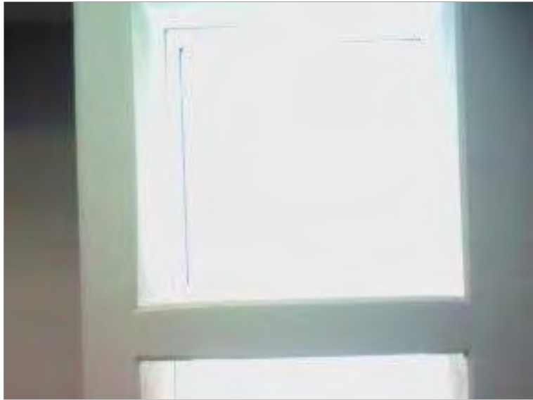
Photo 73: Digital image of the skylights associated with the Ticketing area.
