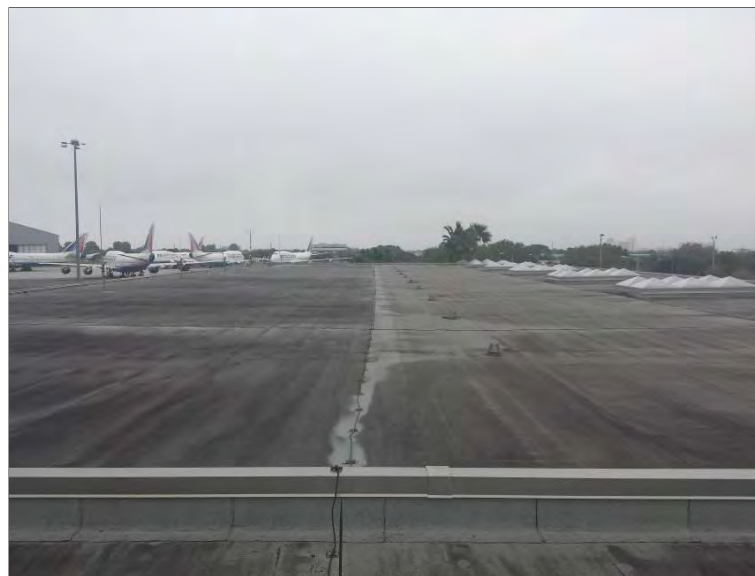
Photo 22: Overview of roof area 19.
