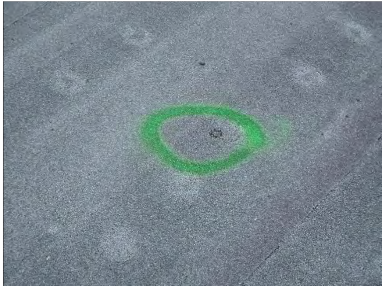
Photo 13: Overview of Thermogram #13 location at Roof #18.
