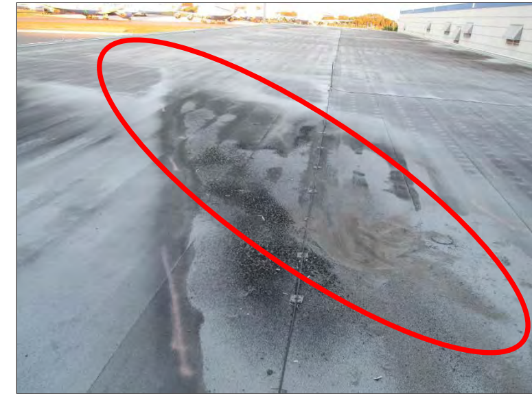
Photo 12: Overview of Thermogram #12 location at Roof #18.
