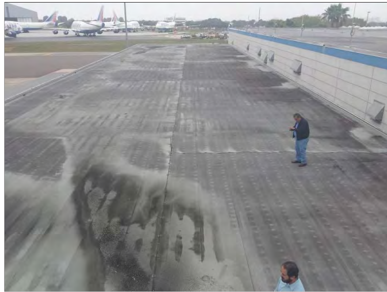
Photo 21: Overview of roof area 18.
