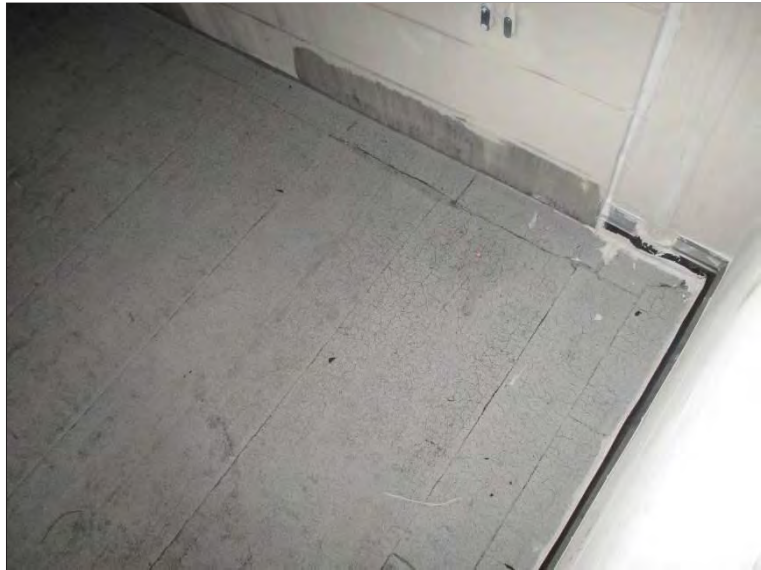
Photo 5: Overview of Thermogram #5 location at Roof #13.
