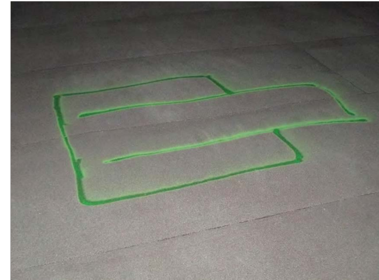
Photo 14: Overview of Thermogram #14 location at Roof #19.
