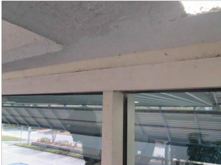
Photo 5: Exterior view of aluminum framed curtainwall systems in the Ticketing area.
