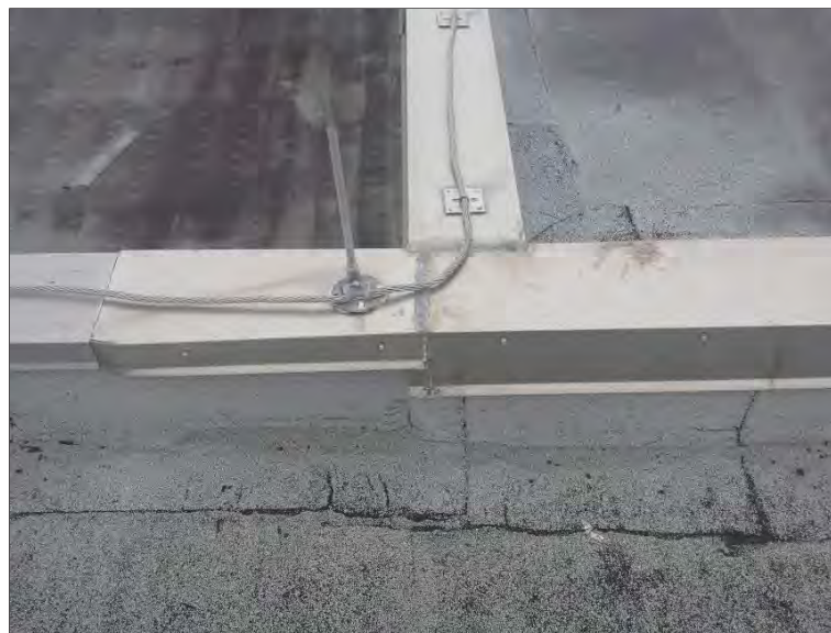
Photo 26: Overview of typical parapet coping and lightning protection.
