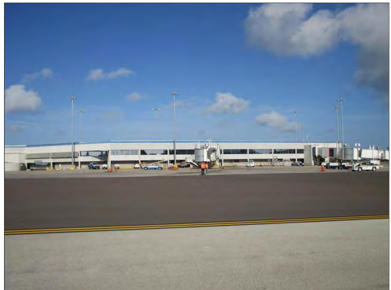
Photo 46: Window assemblies in the Concourse area throughout the east elevation where PSI performed a visual curtainwall and glazed openings survey to document current condition and note observed deficiencies.
