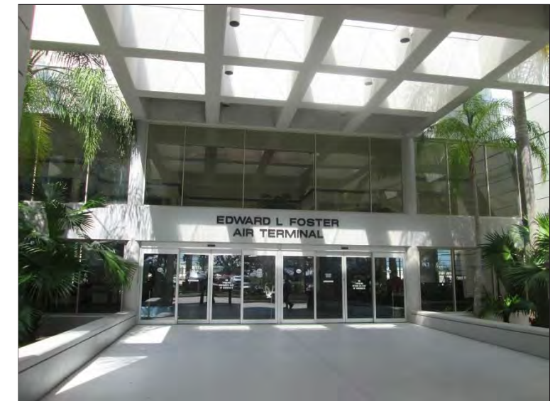
Photo 20: Window assemblies in the Atrium area throughout the south elevation where PSI performed a visual curtainwall and glazed openings survey to document current condition and note observed deficiencies.
