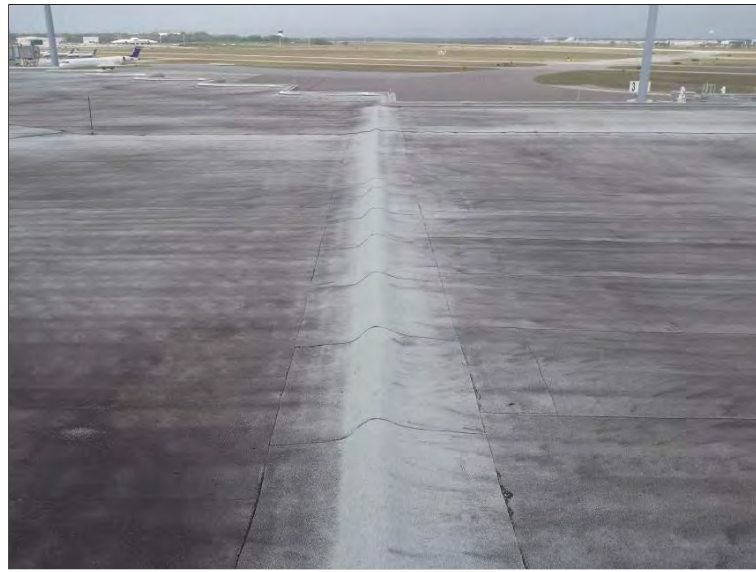
Photo 25: Overview of expansion joint between roofs 20 and 25.
