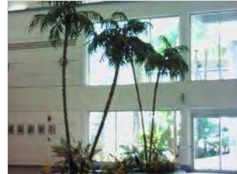
Photo 71: Digital image of the curtainwall systems on the south elevation of the Atrium area.
