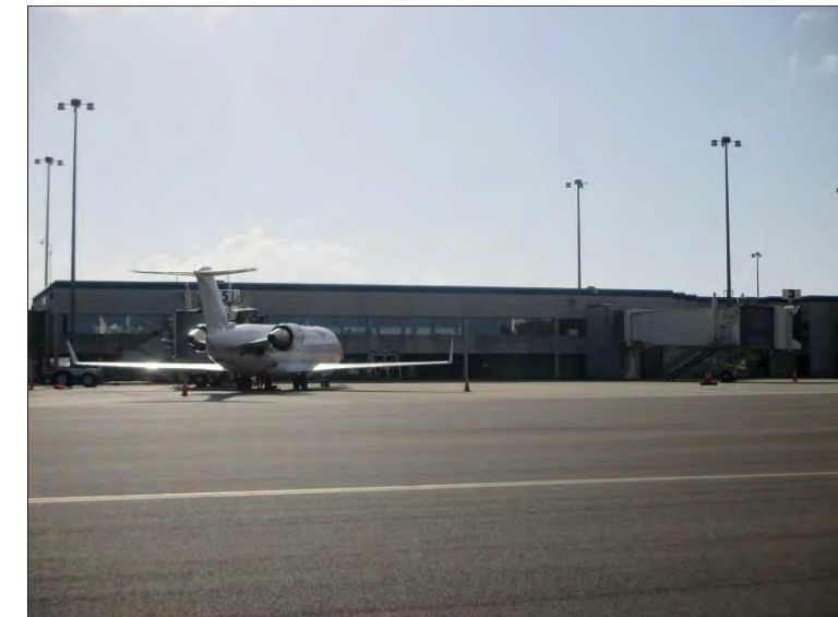
Photo 48: Window assemblies in the Concourse area throughout the west elevation where PSI performed a visual curtainwall and glazed openings survey to document current condition and note observed deficiencies.
