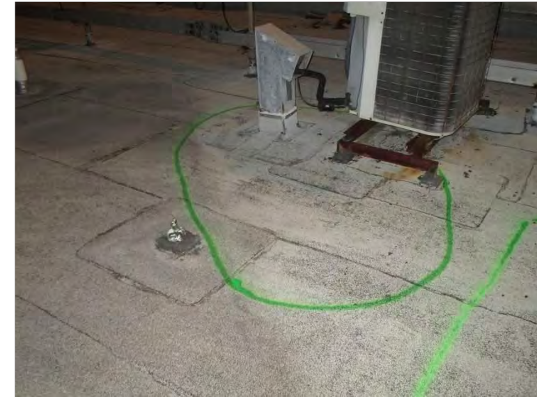
Photo 6: Overview of Thermogram #6 location at Roof #14.
