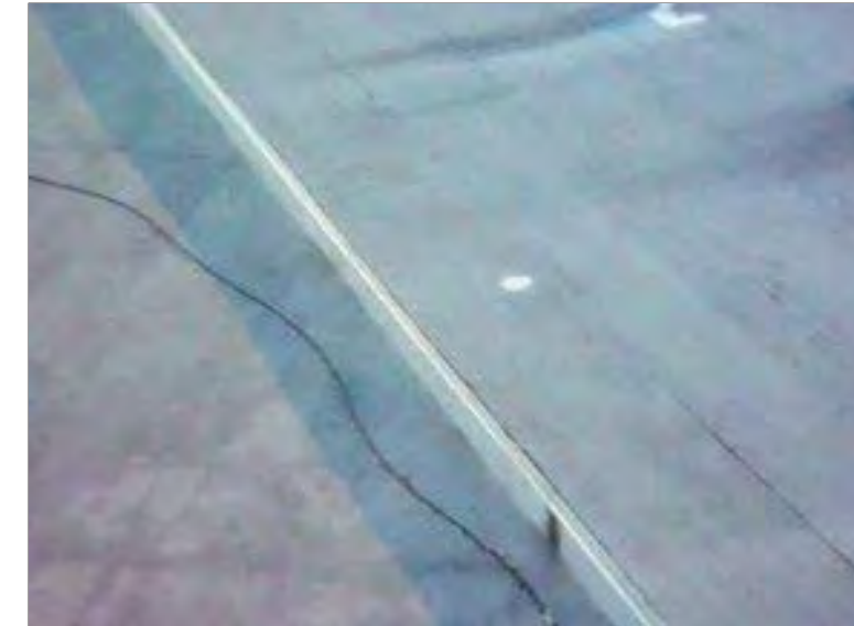
Photo 4: Overview of Thermogram #4 location at Roof #10.
