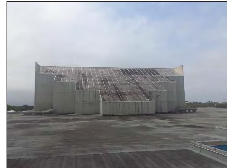
Photo 20: Overview of roof area 16.
