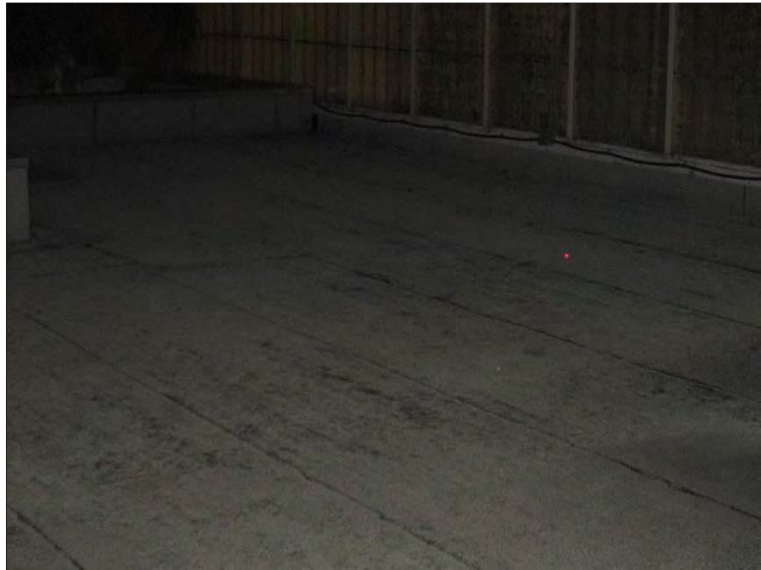
Photo 9: Overview of Thermogram #9 location at Roof #16.
