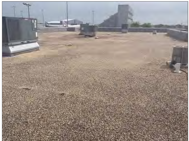
Photo 18: Overview of roof area 5.
