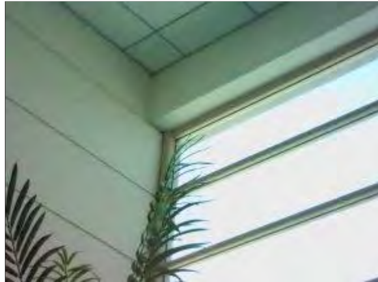
Photo 69: Digital image of the curtainwall systems on the north elevation of the Atrium area.
