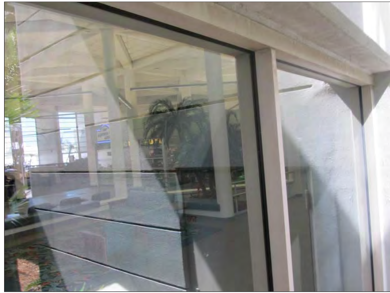
Photo 25: Exterior view of aluminum framed curtainwall systems in the Atrium area.
