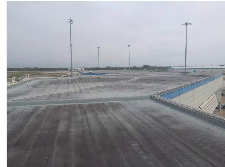
Photo 23: Overview of roof areas 26 and 25 and 20.
