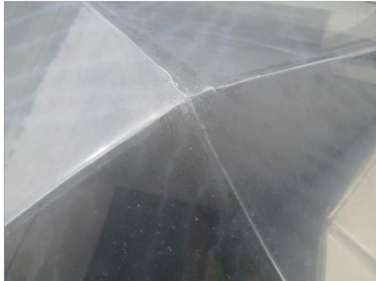
Photo 13: Example of a skylight observed to be in fair condition.
