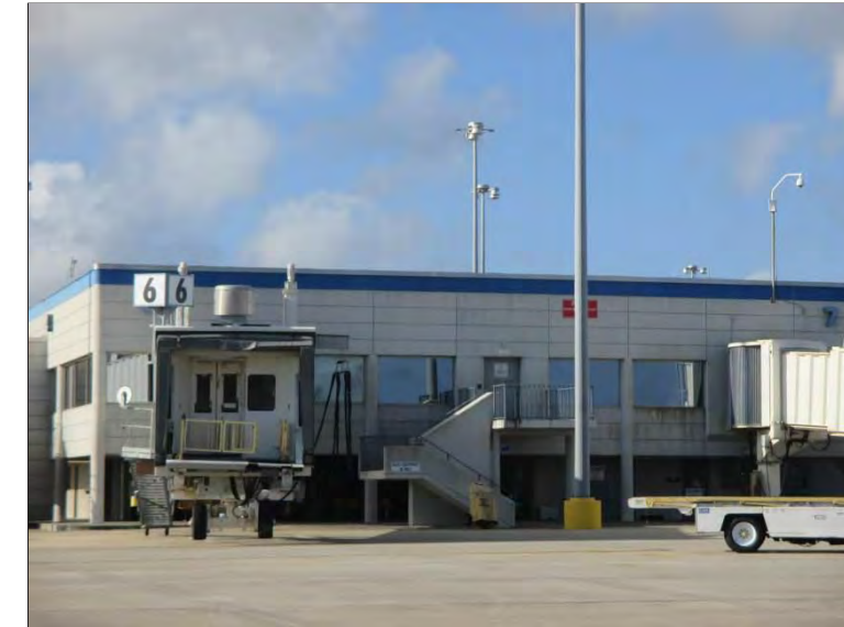
Photo 47: Window assemblies in the Concourse area throughout the north elevation where PSI performed a visual curtainwall and glazed openings survey to document current condition and note observed deficiencies.
