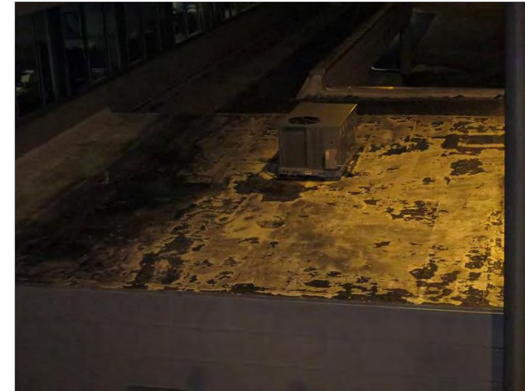
Photo 8: Overview of Thermogram #8 location at Roof #7.
