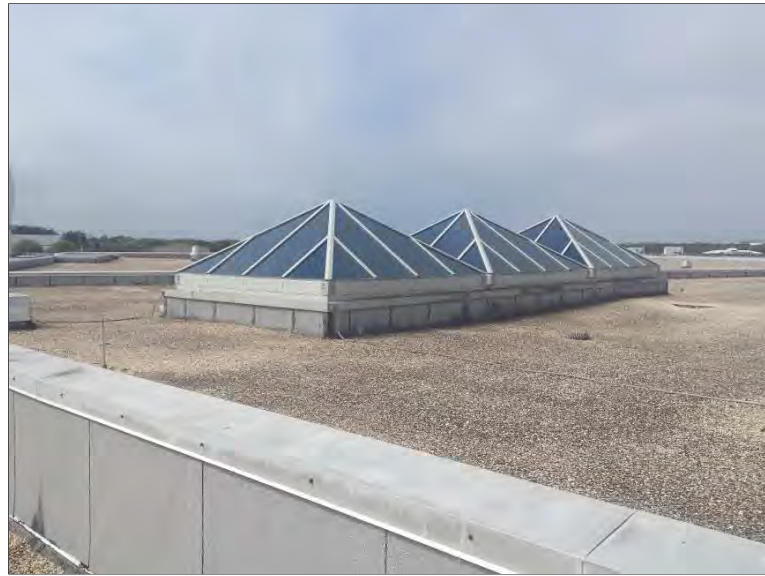
Photo 17: Overview of roof areas 1, 2 and 3.
