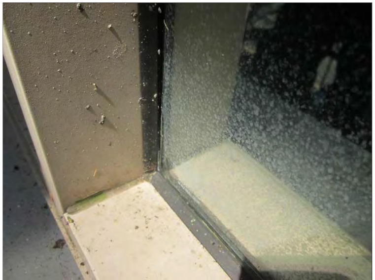
Photo 6: Exterior rubber glazing gasket sealants in the Ticketing area.
