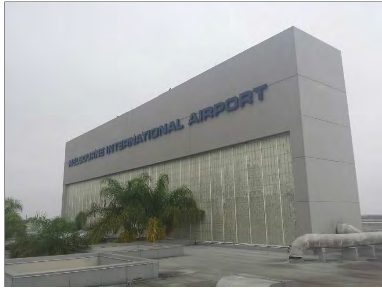
Photo 21: Overview of south elevation of translucent panel system of elevated structure on Atrium roof.
