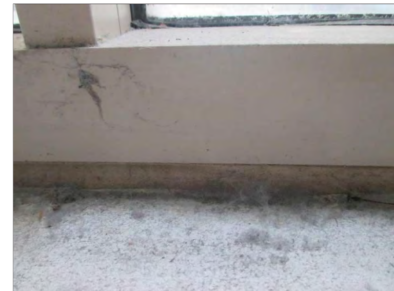
Photo 28: Interior view of the aluminum framed curtainwall systems constructed with interior rubber glazing gasket sealants and flexible perimeter sealant in the Atrium area.
