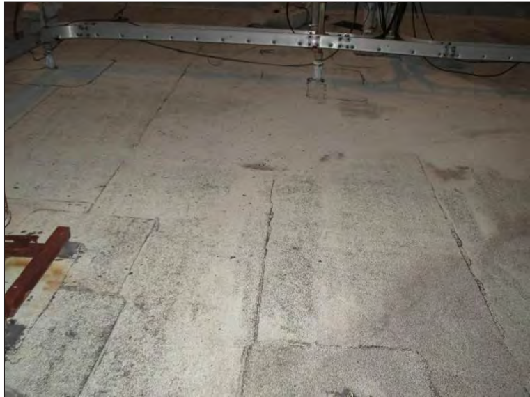
Photo 7: Overview of Thermogram #7 location at Roof #14.
